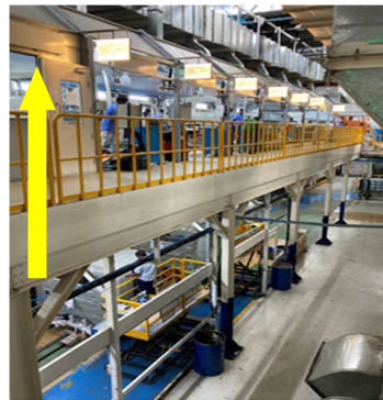
New Topcoat line in Mezzanine floor
