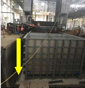
PTED tanks at 4 mtr depth pit
